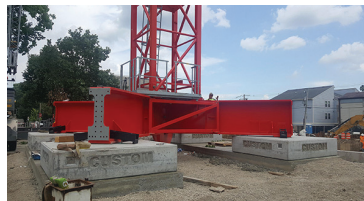
6-8 meter base on concrete engineered mats
