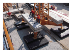
14'9" base on engineered mats Heights up to 177'
