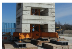
12'5" base on engineered mats Heights up to 137'
