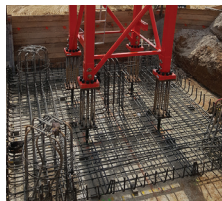
Embed bolt foundation
